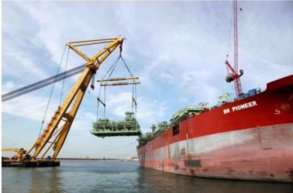
Module Lift onto FPSO
