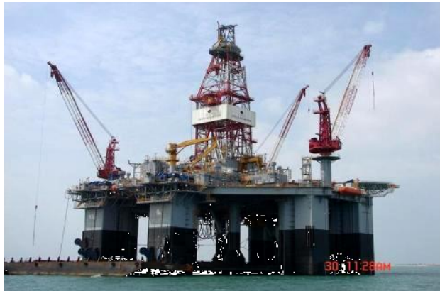
Ocean Endeavor Diamond Offshore Drilling
